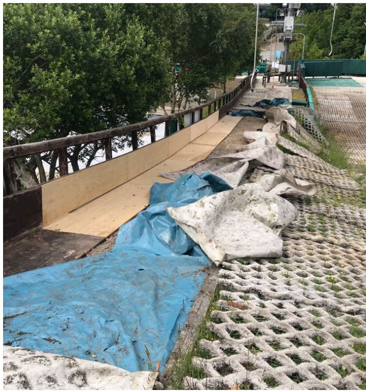
Above: Repairs have been made to the Poma lift track on the Intermediate/middle slope and large sections of new white Dendix matting have been installed on the main slope
